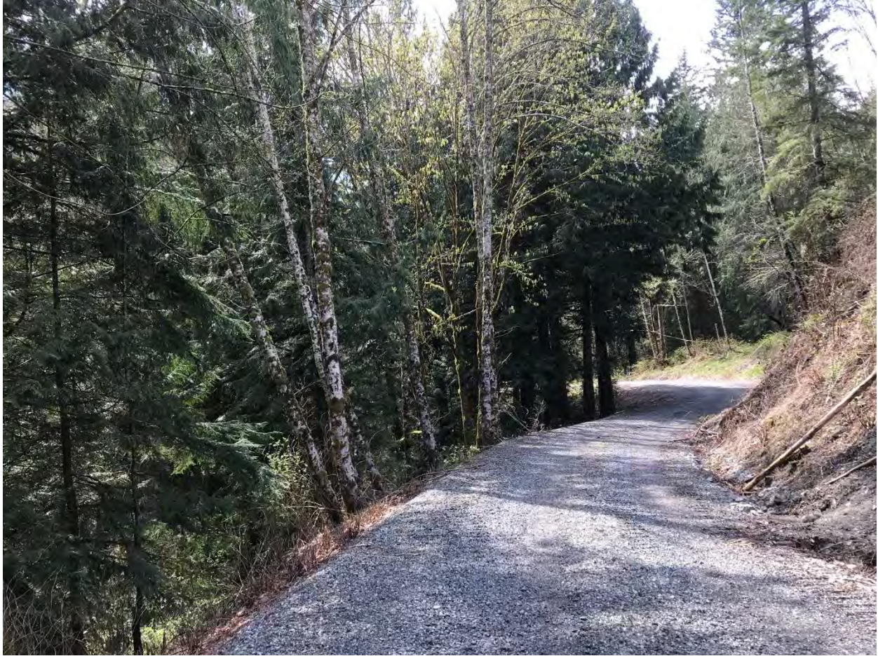
Private internal Haul Road. Around corner in distance is private bridge.
